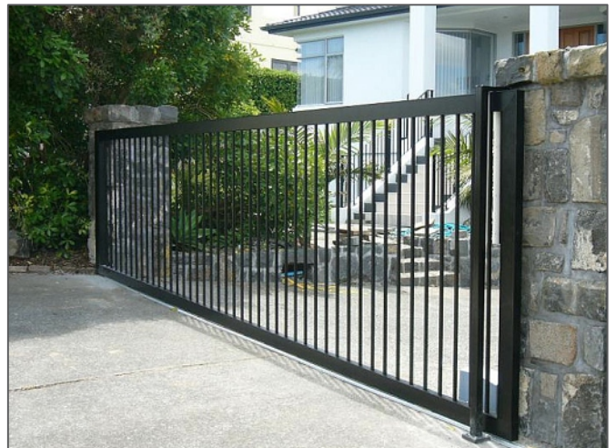
Vehicle access Gate, Sliding with Baluster infill.
