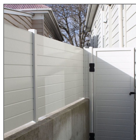
Pedestrian Gate, horizontal T&G Slat. Fence on Nib Wall same infill
