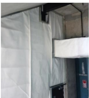
Fire Escape Stairwells- Civic Centre Christchurch
