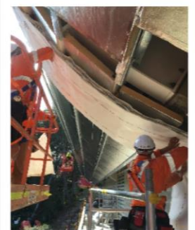
Curved External Wall - Aquatic Centre NSW
