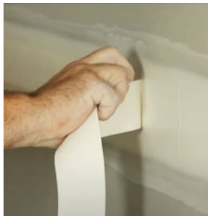
First Coat - Taping
