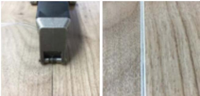
Groove just through the wear layer and into the white backing taking an even piece from each side of the seam/ cross join.
