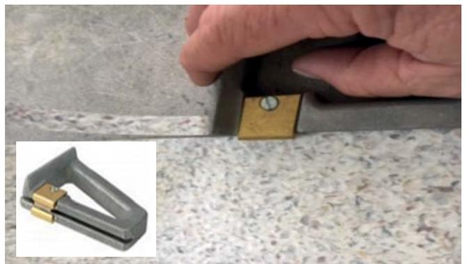
Scribe the seams using Armstrong Flooring S-83 Recess Scriber set to provide a maximum gap of 0.4mm.
