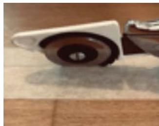
Insert the needle and allow the seam sealer to flow into the seam as the needle moves along, do not rush this part. The seam will push apart and back together allowing the seam sealer to melt the wear layer fusing the two together.
