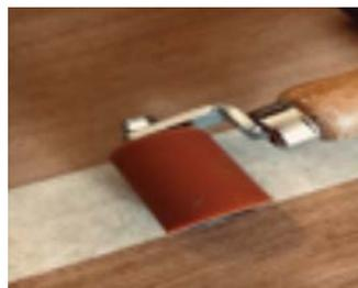
Cover the seam / cross join using a quality masking tape, roll the tape to achieve good contact to the PU coating. Using a rolling knife down the seam /cross join to split the tape.
