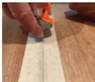
Allow approximately 20 minutes before removing the masking tape taking away any excess seam sealer.
