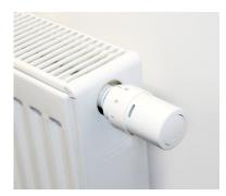
The radiator valve (TRV) allows for individual temperature control on each radiator
