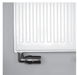
— The radiator valve (TRV) allows for individual temperature control on each radiator
