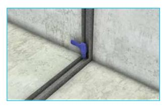
Then use the fixings to secure the C-track.
