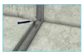
If the surrounding surface is uneven or if you're not sure you have a good seal, add a continuous bead of sealant around the perimeter of the C-track where it contacts the surrounding surface.
