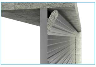
Angle is then fixed to the soffit at 400 mm centres, then fixed to the panel at 400 mm centres.
