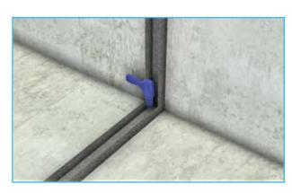
Then use the fixings to secure the C-track.
