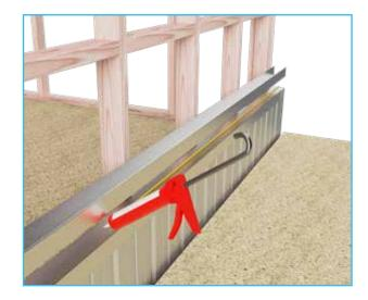
Place bead of fire sealant into the internal corner of the top C-track.
