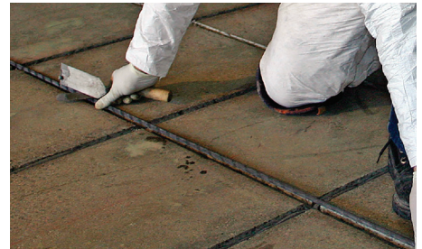
Near-Surface-Mounted FRP Reinforcement
