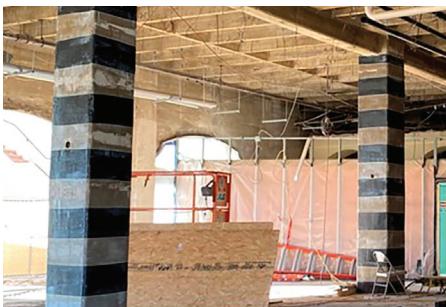
Column Shear Strengthening
