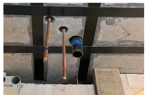
Slab Penetration Flexural Strengthening
