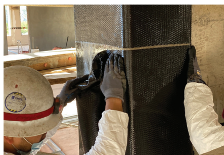
Boundary Element Confinement
