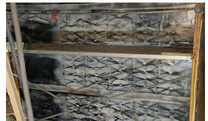
Wall Strengthening with FRP Anchors
