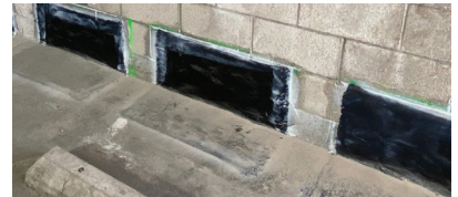
Slab-to-CMU Wall Joint Shear Strengthening
