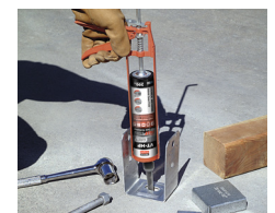
Threaded Rod Anchoring
