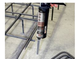
Rebar Doweling
