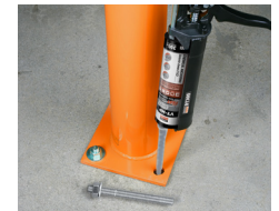
Threaded Rod Anchoring
