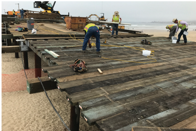
Docks, Pier's, Boardwalks, Jetty and Wharf construction
