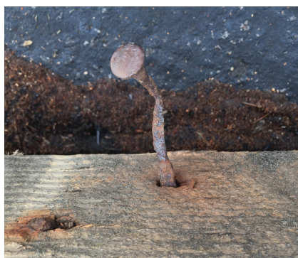
The effect of corrosion on HDG spikes
