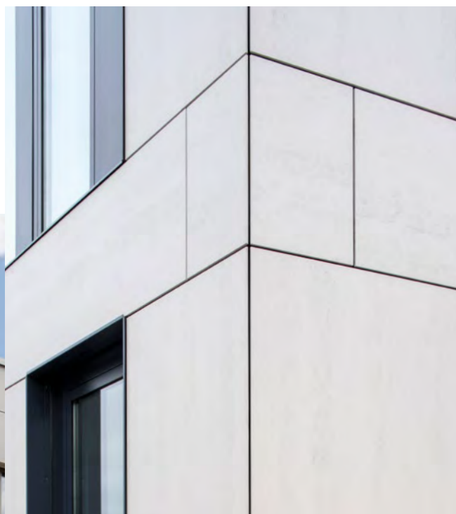
Shittethelm Office Building (Germany)
