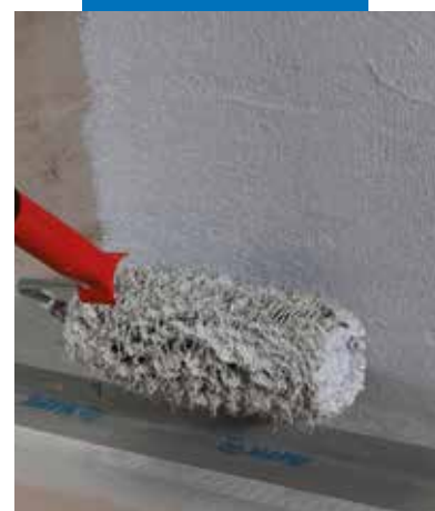
Application of Mapegum WPS with a roller
