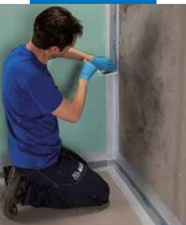
Application of Mapeband PE 120 using Mapegum WPS
