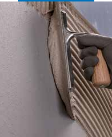
Installing floor covering using Ultramastic III
