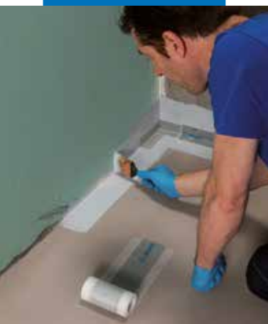
Application of Mapeband PE 120 using Mapegum WPS
