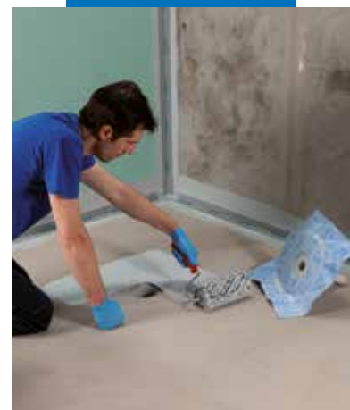
Application of a Drain Vertical fitting using Mapegum WPS
