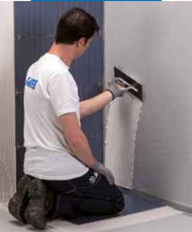
Installing wall covering using Keraflex Maxi S1
