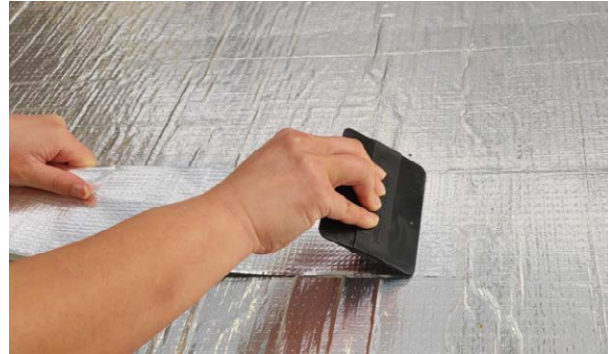
Figure 2. Applying pressure as the tape is being rolled out will achieve maximum adhesion.
