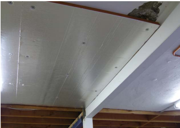
Figure 6. Penetration example - Kooltherm K10 G2 Soffit Board installed tight around the fire collar and HDPE service pipe.
