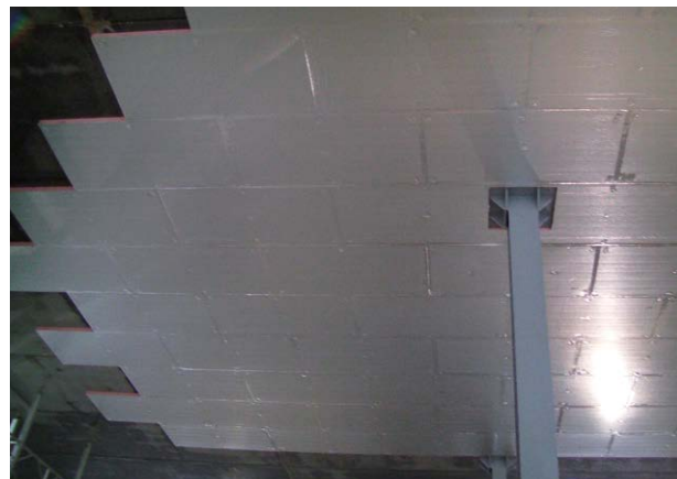
Figure 4. Board joints staggered.
