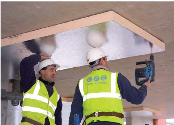
Figure 5. Board joints squared.
