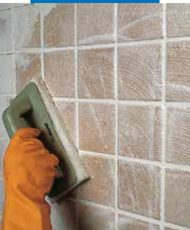
Finishing of single fired tile wall with a Scotch-Brite® pad
