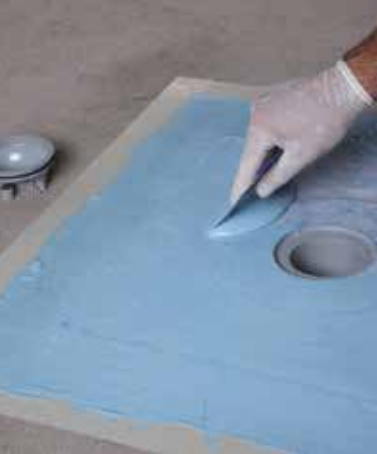
Impregnating Drain Vertical fabric with Mapelastick AquaDefense
