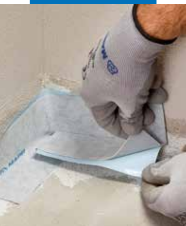
Application of Mapeband SA in corners
