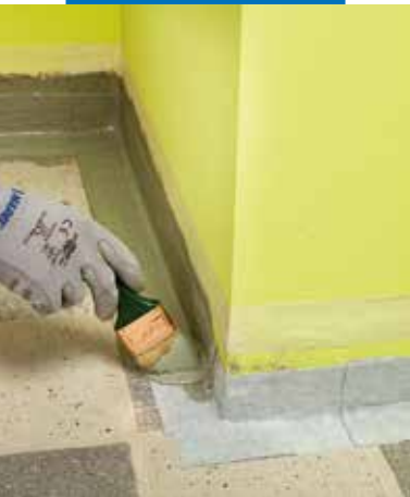
Application of Mapeband SA on a screed
