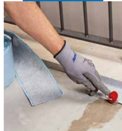
Application of Mapeband SA around edges
