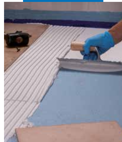
Bonding tiles on Mapelastac AquaDefense
