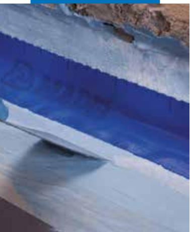
Application of Mapeband on a wall-floor fillet joint with Mapelastick AquaDefense
