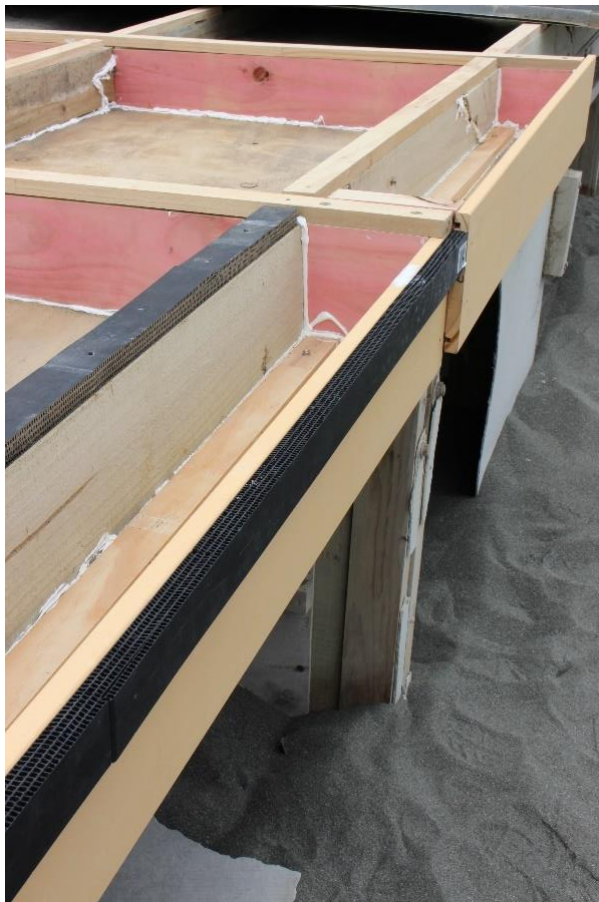
Figure 4. Vent opening on the seaward side of the structure.
