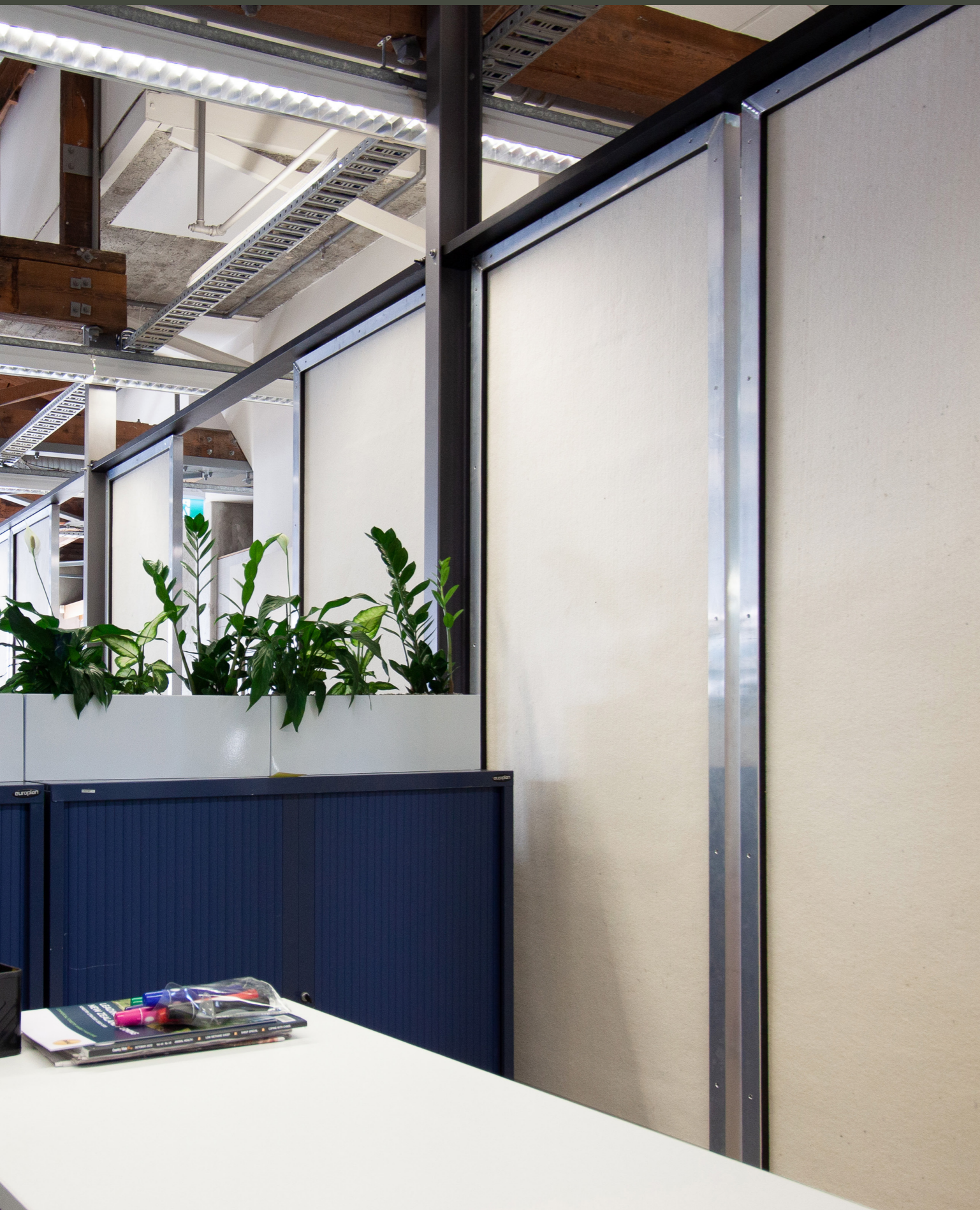
Floc Panel installed at Pāmu, Wellington.
