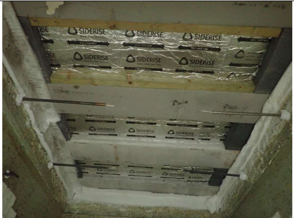
The exposed face of the floor assembly prior to testing
