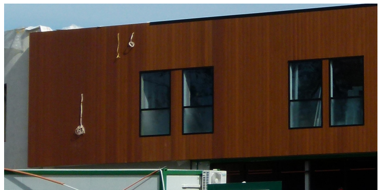
Incorrectly Mixed batches and boxes, leaving blocks of colour
