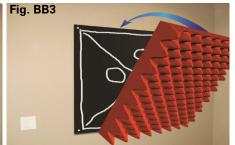
STEP 3 Firmly push the panel onto the backing board, making sure that even pressure is applied to all areas that the adhesive has been applied to.
