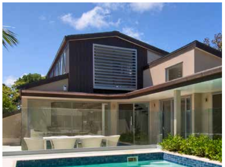
MOTORISED, VERTICAL SUN LOUVRES INCLUDING STRUCTURAL FRAME
