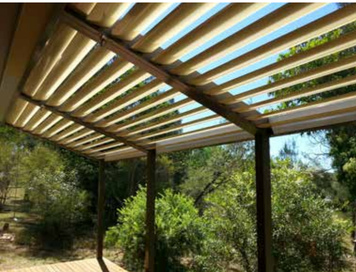
HAND ADJUSTABLE, OVERHEAD SUN LOUVRES FITTING WITHIN AN OPENING
