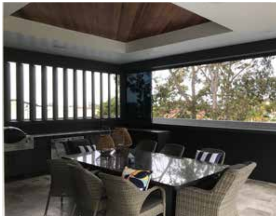
VERTICAL SUN LOUVRES FITTED INTO A FRAME
