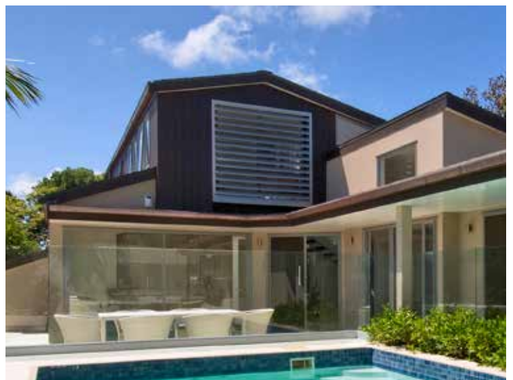
MOTORISED, VERTICAL SUN LOUVRES INCLUDING STRUCTURAL FRAME
