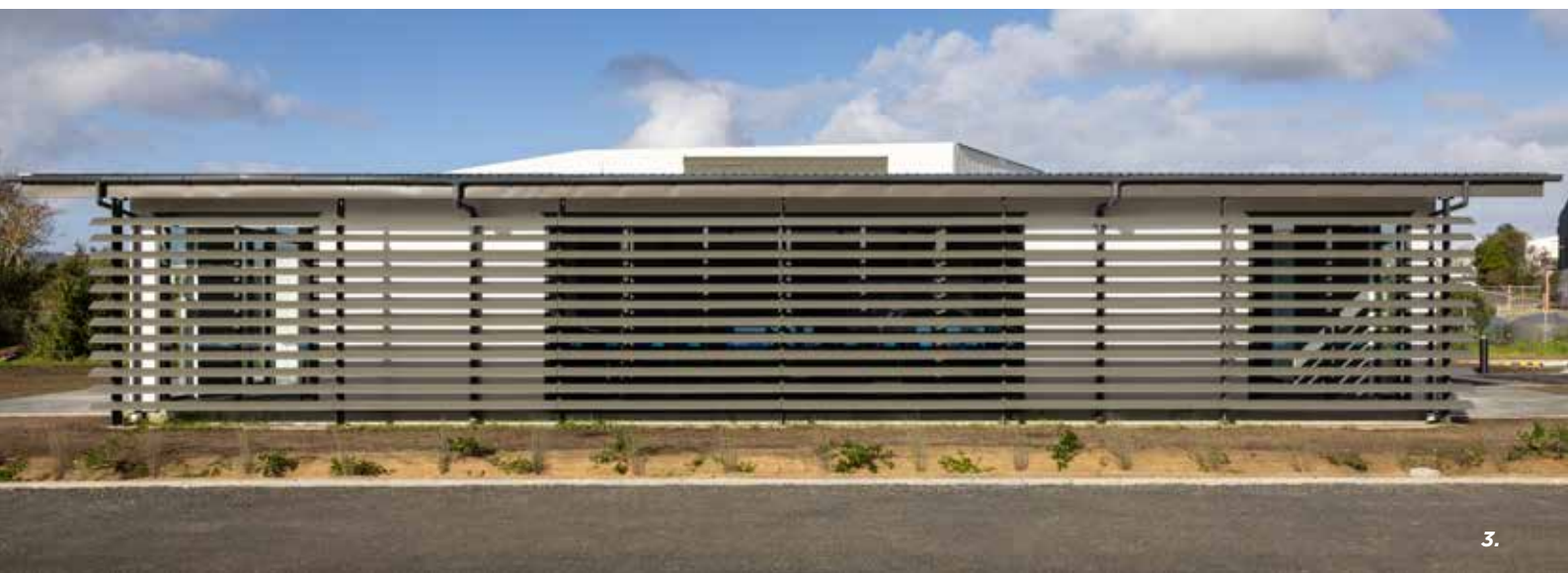
1. BRACKET FIXED 120MM AIRFOIL LOUVRES 2. BRACKET FIXED RL300 MITRE LOUVRES 3. BRACKET FIXED 150MM MIDI LOUVRES
