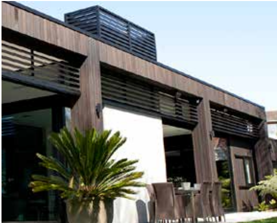
END FIXED CHIMNEY SURROUND, AUCKLAND
