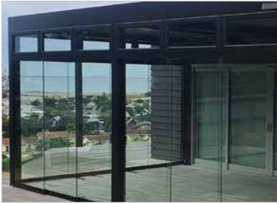
OVERHEAD RECTANGULAR PANELS
