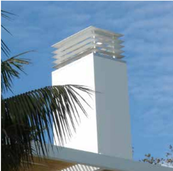
BRACKET FIXED CHIMNEY SURROUND WITH MITRED CORNERS
