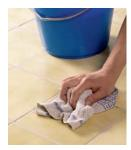
Mount the new tiles on the adhesive. Joint the tiles and let the floor dry for two weeks before turning on the heating.
