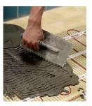
Before laying the self-adhesive mat, your existing floor should be clean and dry and primed if necessary. Once the mat has been tested, it can be rolled out and laid on the floor.
