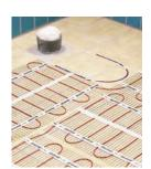
Then cut a 10 mm wide groove into the floor and wall for the floor sensor and tube. The tube allows for easy removal of the floor sensor, if required. Glue the tube housing the floor sensor into the channel and seal the end of the pipe with duct tape.
