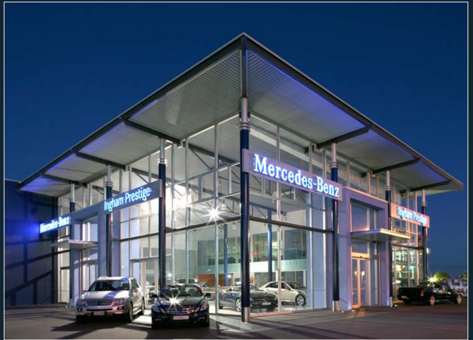
Exterior circular columns braced the façade against lateral movement.
