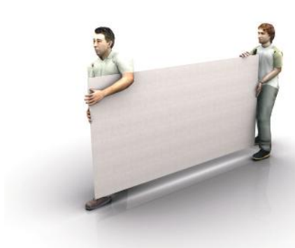
Figure 3 Always carry the panel on edge but DO NOT store on edge
